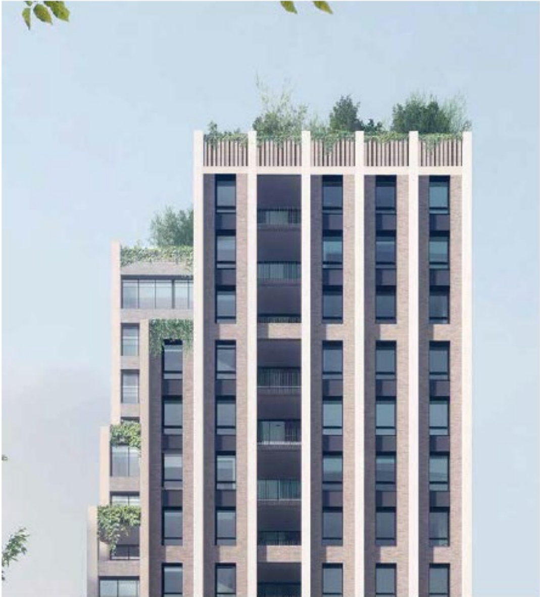
Figure 23 Off-form concrete lintels to provide clear delineation at the top of the façade, also material changes to brickwork for the elevational treatment of the tower
