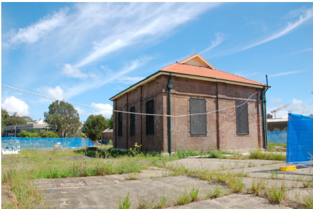
Figure 3 Valve House viewed looking south-west (Source: Heritage Brief prepared by GBA Heritage at Appendix 15)
