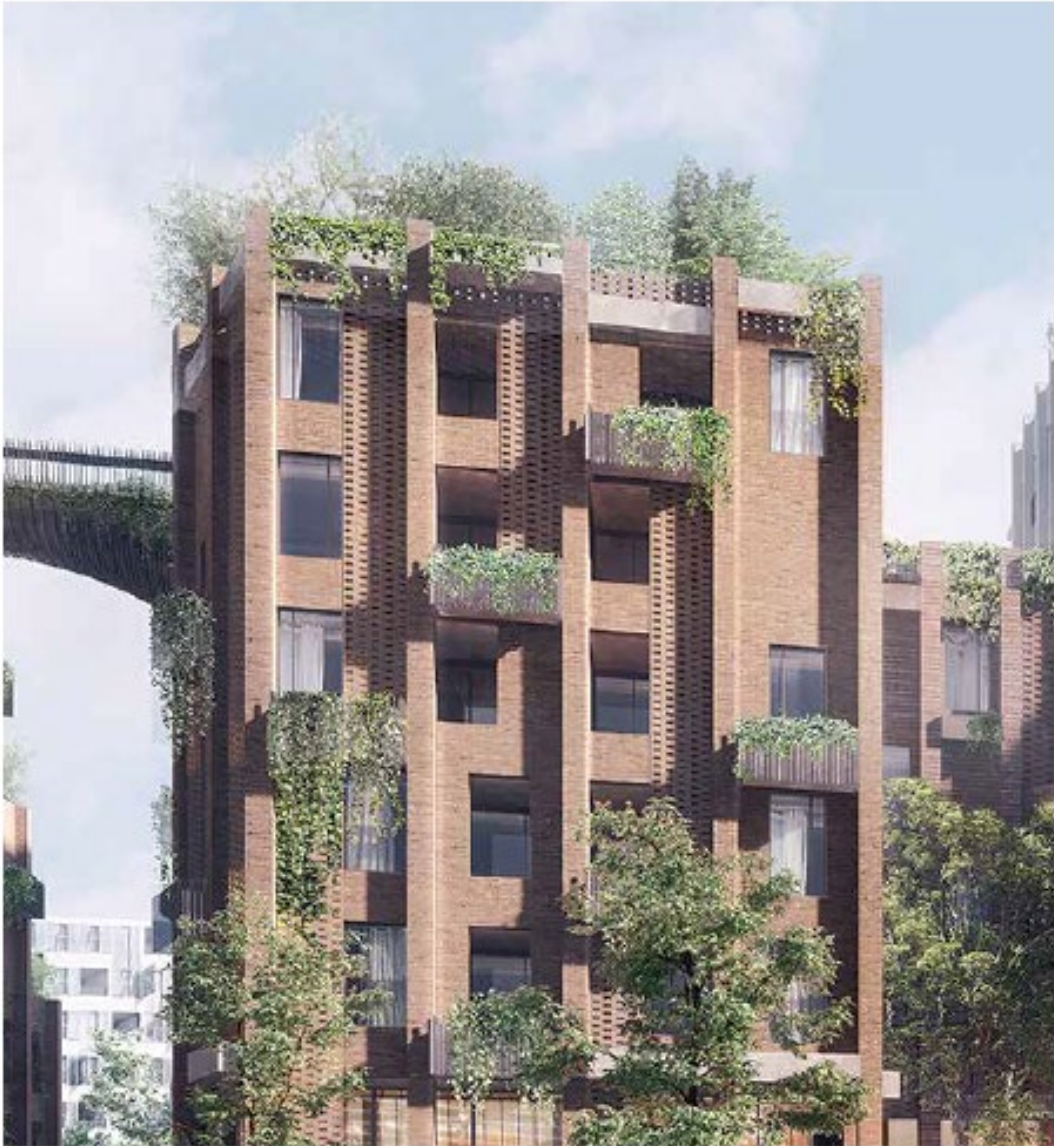
Figure 22 Off-form concrete lintels to provide clear delineation at the top of the facade
